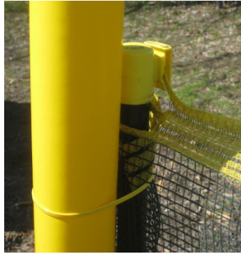
Foul pole secured to fence end pole
