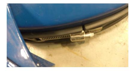
Position the clamp so you have room for the screw driver to tighten the band clamp.
