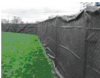
Example of windscreen not installed properly
