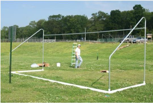
Attach rear crossbar into tee fittings on backstays. Use hardware detailed on assembly drawing. Now tighten all hardware. With goal in the face down position attach the net using the “*Easy Clip*” net attachment system. If the net is installed in this position, there is no need to climb a ladder and attach netting. Once complete, move the goal into the playing position. **Repeat for the other side.**
