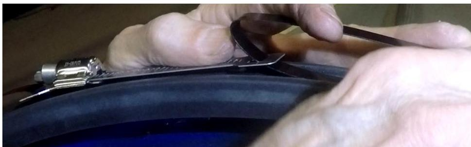
19. Tighten until band is secure.
